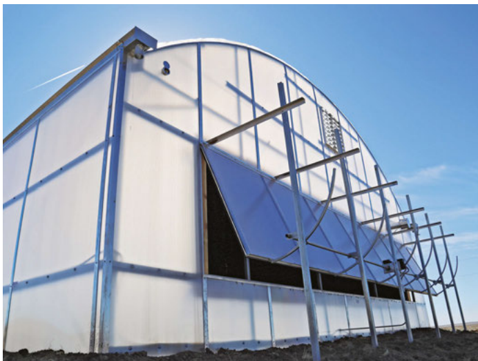
Opening side vents on a greenhouse helps ventilate the space. (Photo courtesy of GrowSpan Greenhouse Structures.)
